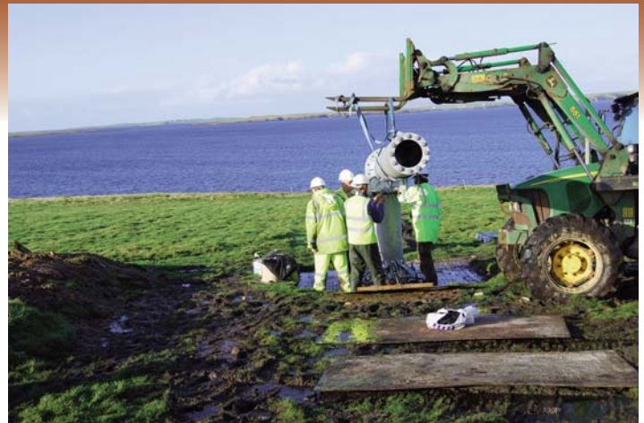
Wind turbine installation
