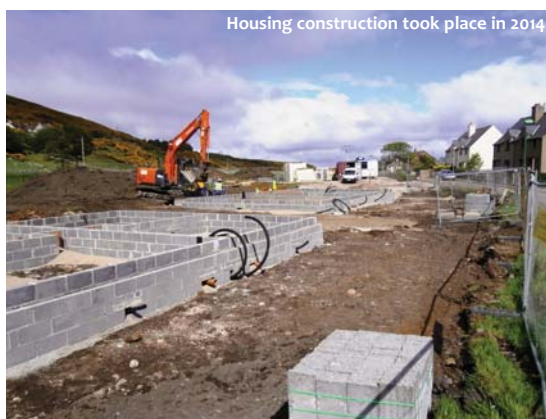
Housing construction took place in 2014
