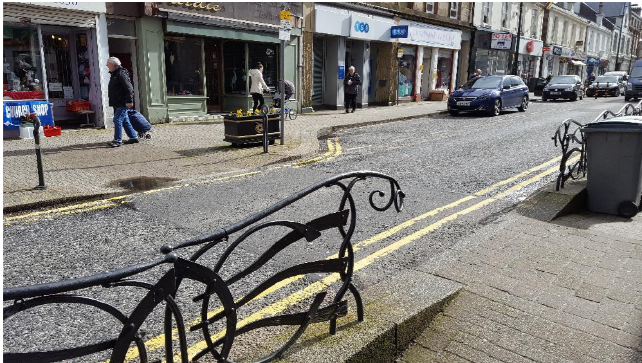
Lack of tactile paving at crossing points
