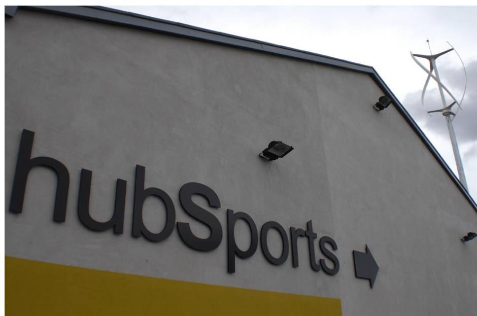
Ground source heat pump and small wind turbine Wellhouse Hub Sports, Glasgow
