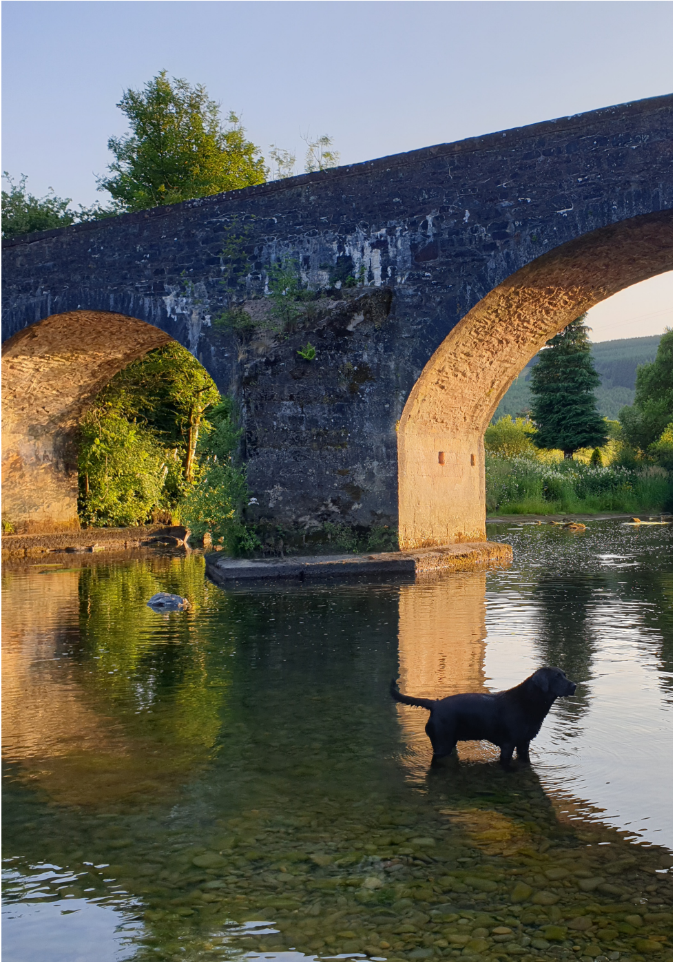
The Bridge at Bentpath
