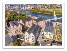
Given the changes in working environments post-Covid, the flat designs include the integration of home/office space. For environment purposes, they also include recycling facilities, photo voltaic panels on the roof, and waste water heat recovery systems. Legislation changed during the process which led to a redesign.
